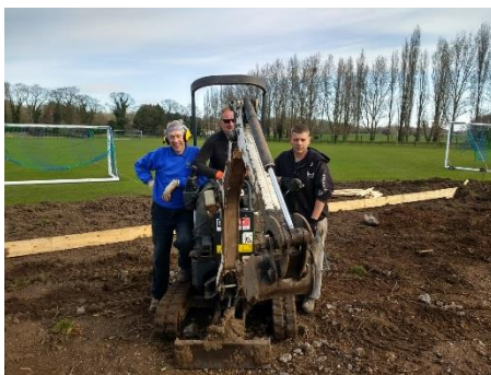
Digging the foundations for the Bowls Pavilion
