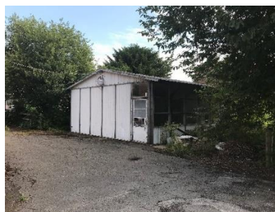
Old Classroom (due for demolition)
