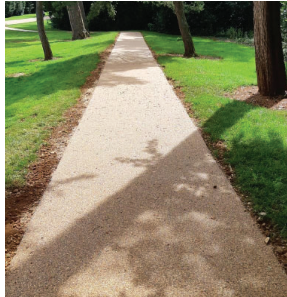
Tar Spray and Chip Approx £19,000
